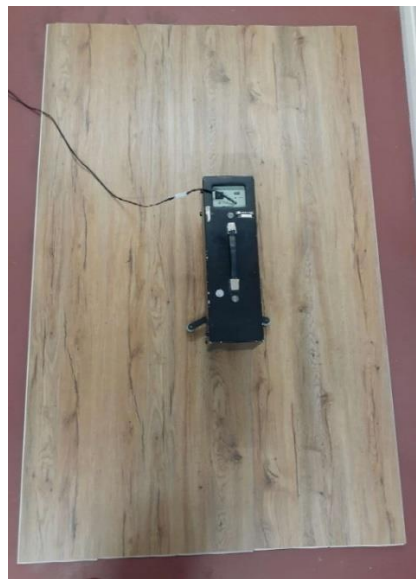
SPC Hybrid plank with 2mm IXPE foam underlay on top of the base floor
